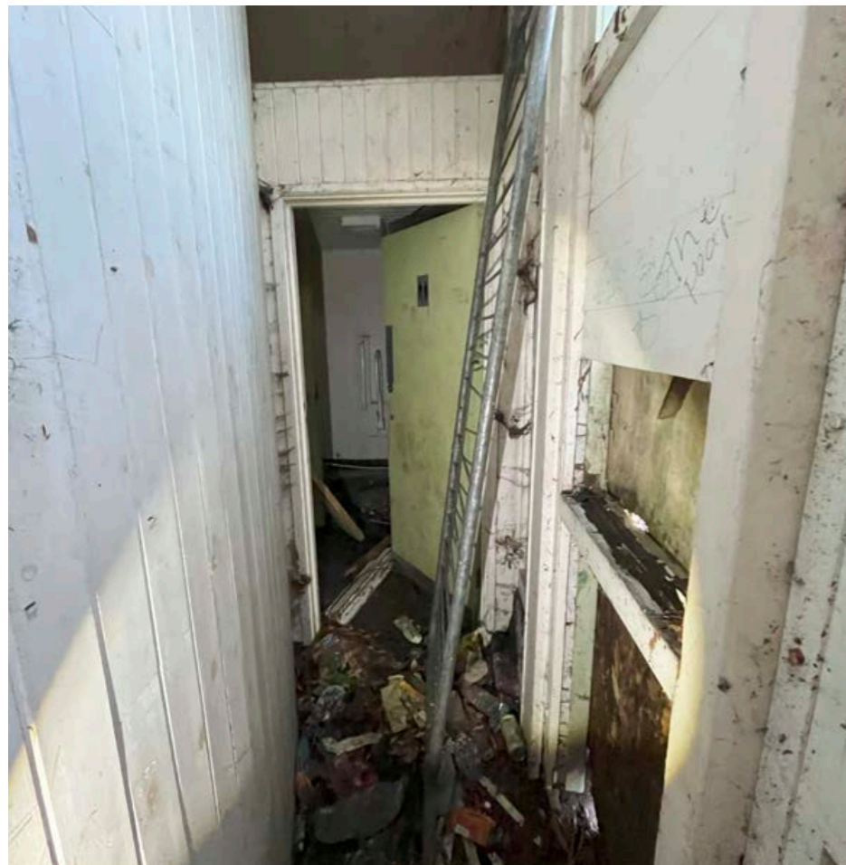
View to lobby space and WC
