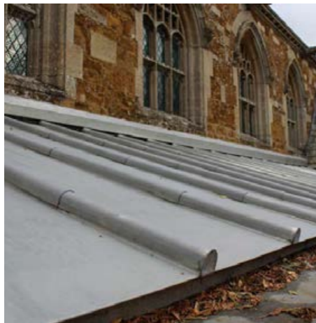
Example of a terne coated stainless steel roof with traditional roll joints, as an alternative to lead. (Historic England)
